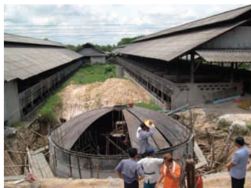
Anaerobic digester for biogas production in a commercial pig farm – Central Thailand 2005
